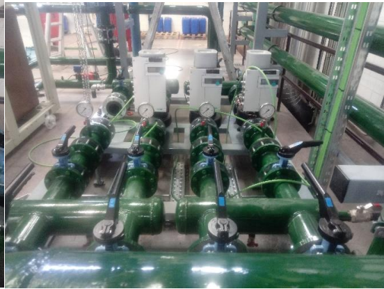
The pictures show the installation process of the thermal energy meter, devices and thermostatic valves
