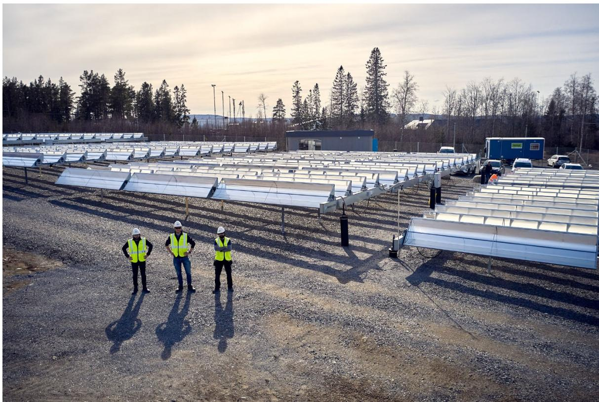
Högslätten Solar Park, located in Härnösand, Sweden, is a large-scale solar district heating facility operated by Absolicon. The Absolicon T160 collectors produce heat with a working temperature range of 73°C to 160°C, and they provide the district heating network supply line with temperatures up to 120°C.
