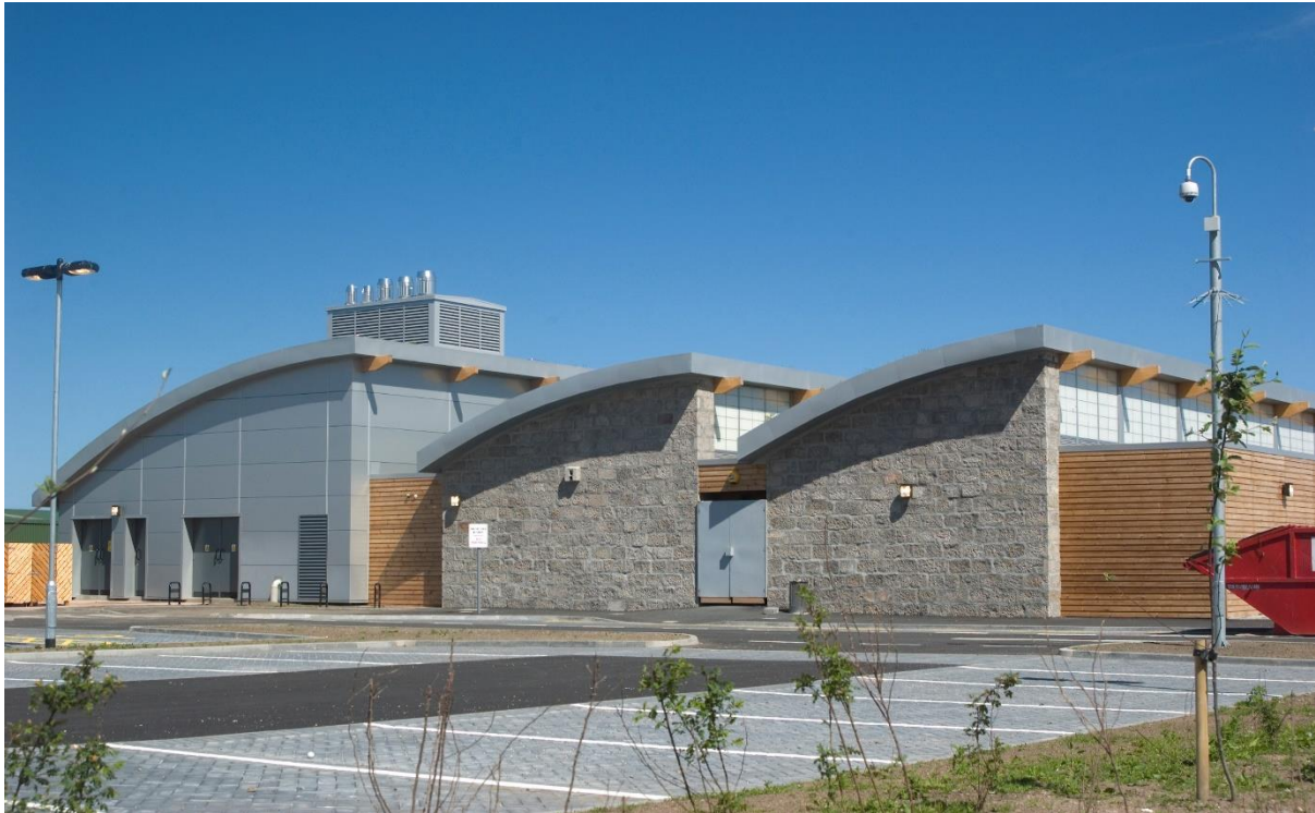
Seaton Energy Centre, Aberdeen
