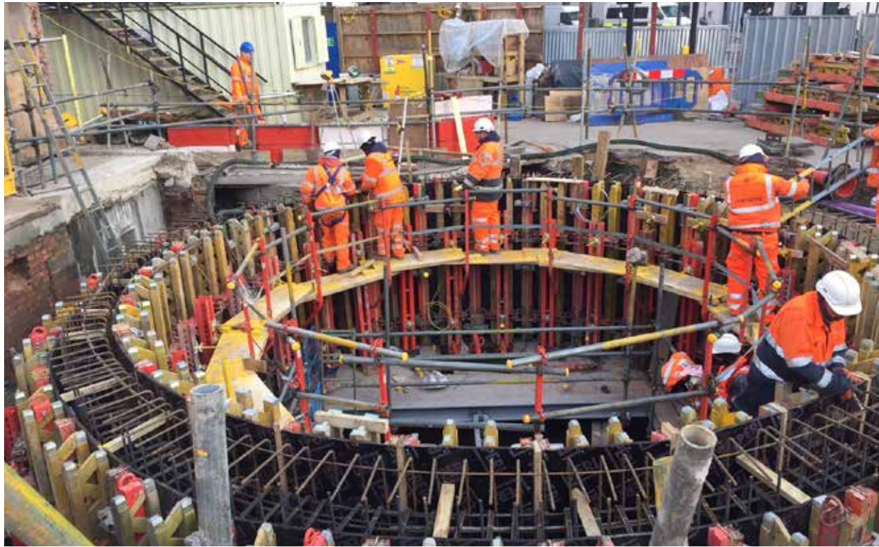
Figure 14. Laying foundations
