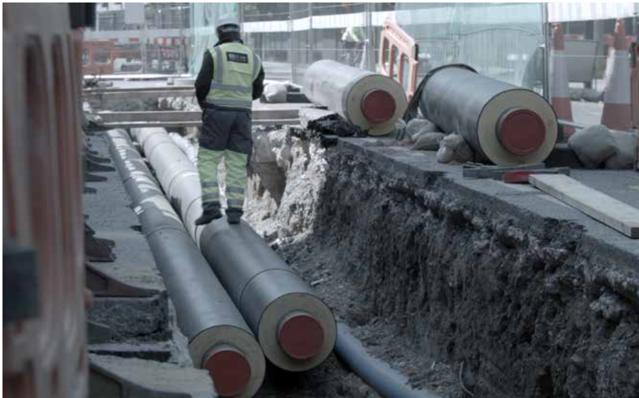
Figure 15. Laying the underground pipe network in Central Street
