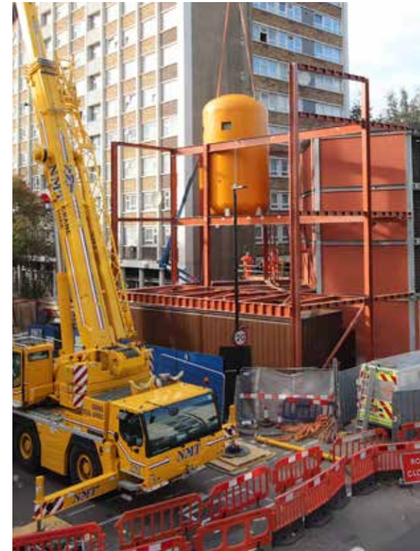
Figure 16. Craning thermal store into the new energy centre
