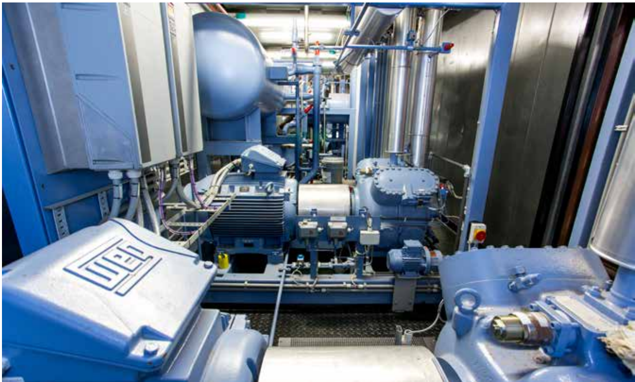
Figure 5. The heat pump in new energy centre
