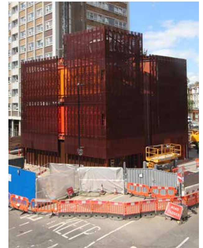
Figure 19. Completed installation of façade panels
