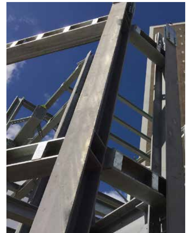
Figure 13. Ventilation shaft steel frame
