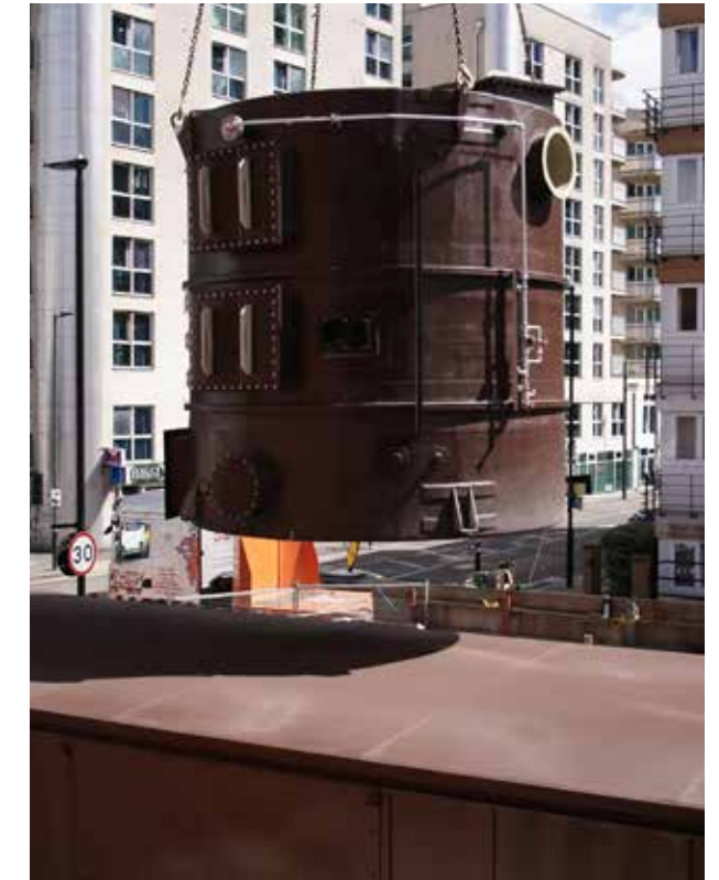
Figure 18. Installing the carbon scrubber
