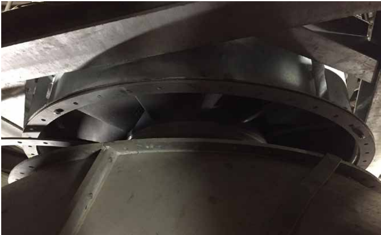
Figure 9. Ventilation shaft fan
