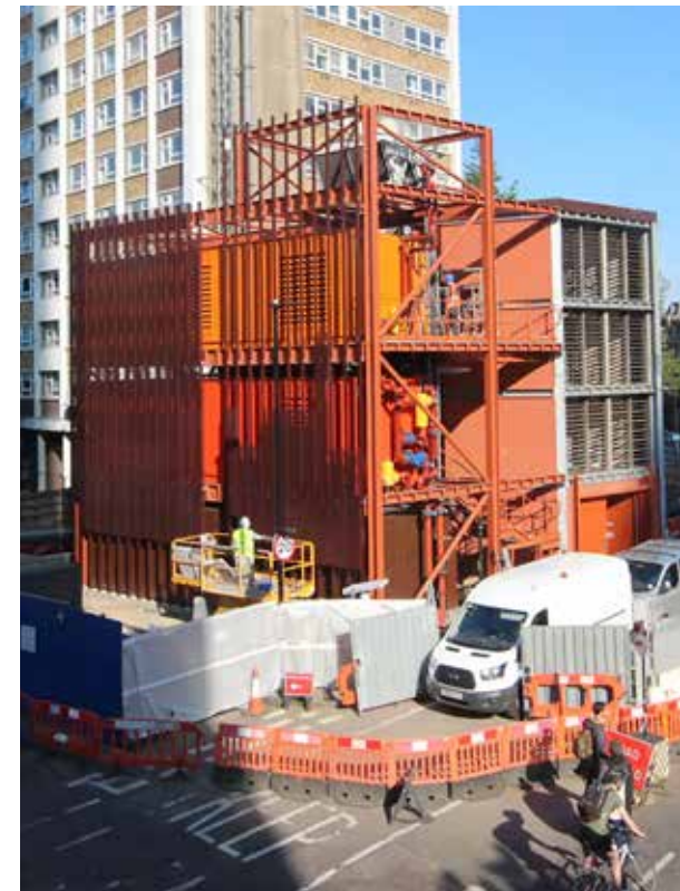
Figure 17. Starting the installation of façade panels
