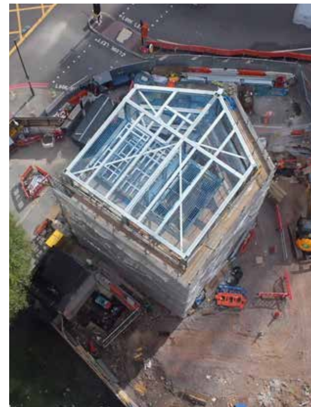
Figure 11. Ventilation shaft head house steel frame
