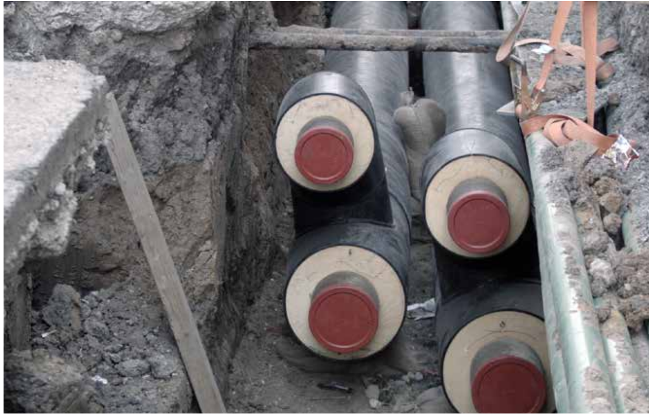
Figure 20. Insulated pipes
