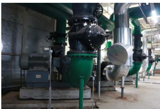
Frozen water pump, cooling water pump
