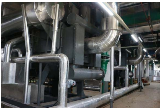
Electric refrigeration unit, lithium bromide refrigeration unit
