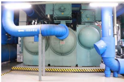
Electric refrigeration unit, lithium bromide refrigeration unit
