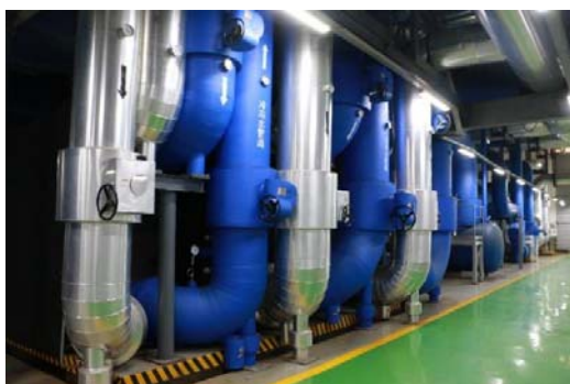
Frozen water pump, cooling water pump
