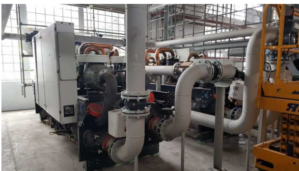
HEAT PUMPS TRANE MODELO RTWF300 HE REFRIGERANT: R1234ze
