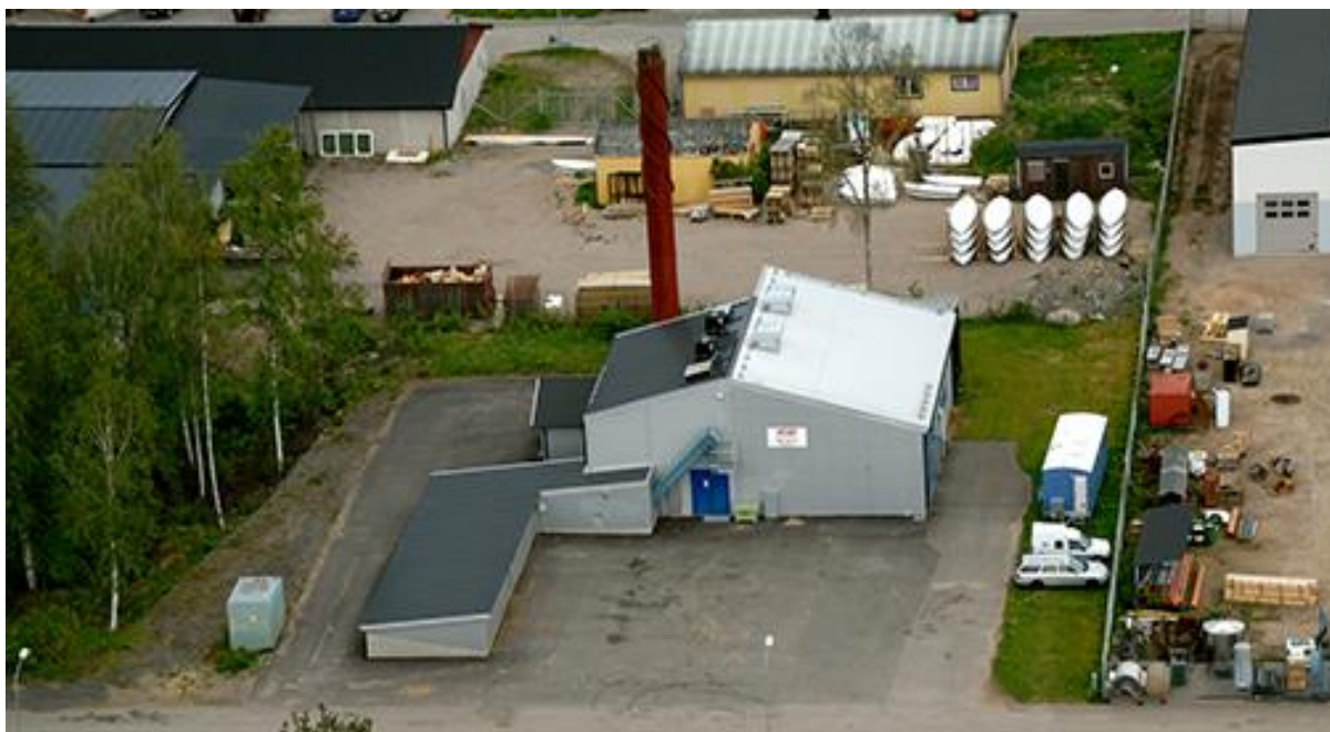
Figure 2: An aerial view of the Rottne district heating production plant
