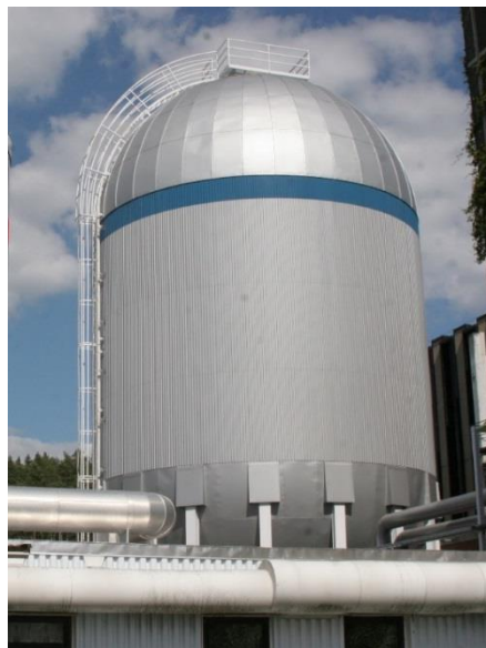
Figure 2. The Accumulator Tank at Sandviksverket in Växjö.
