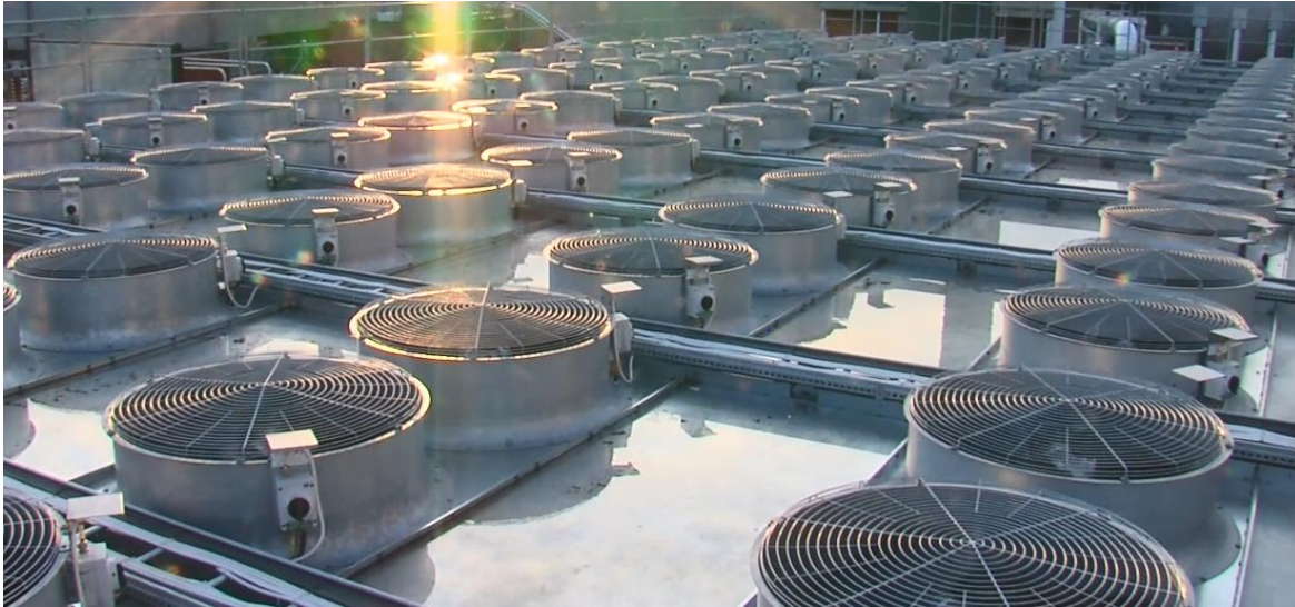
Figure 1. 144 fans on the top of the air-cooled liquid chiller at Sandviksverket in Växjö.
