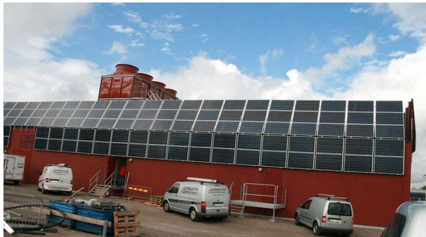
Figure 6. PV-panels at cooling production plant at Västra Mark and the Green Data Centre.
