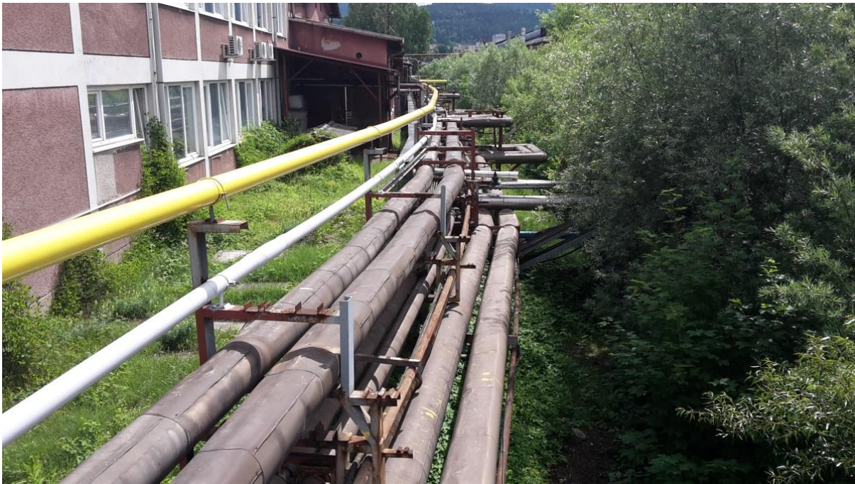
Figure 3: Distribution pipe lines (DN 200)
