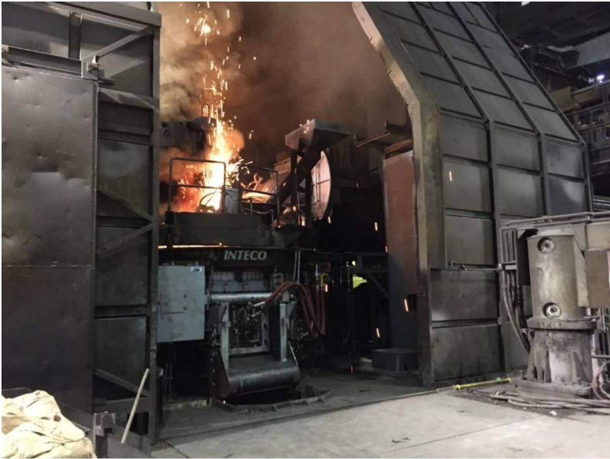
Figure 1: Electric arc furnace (source of waste heat) in SIJ Metal Ravne
