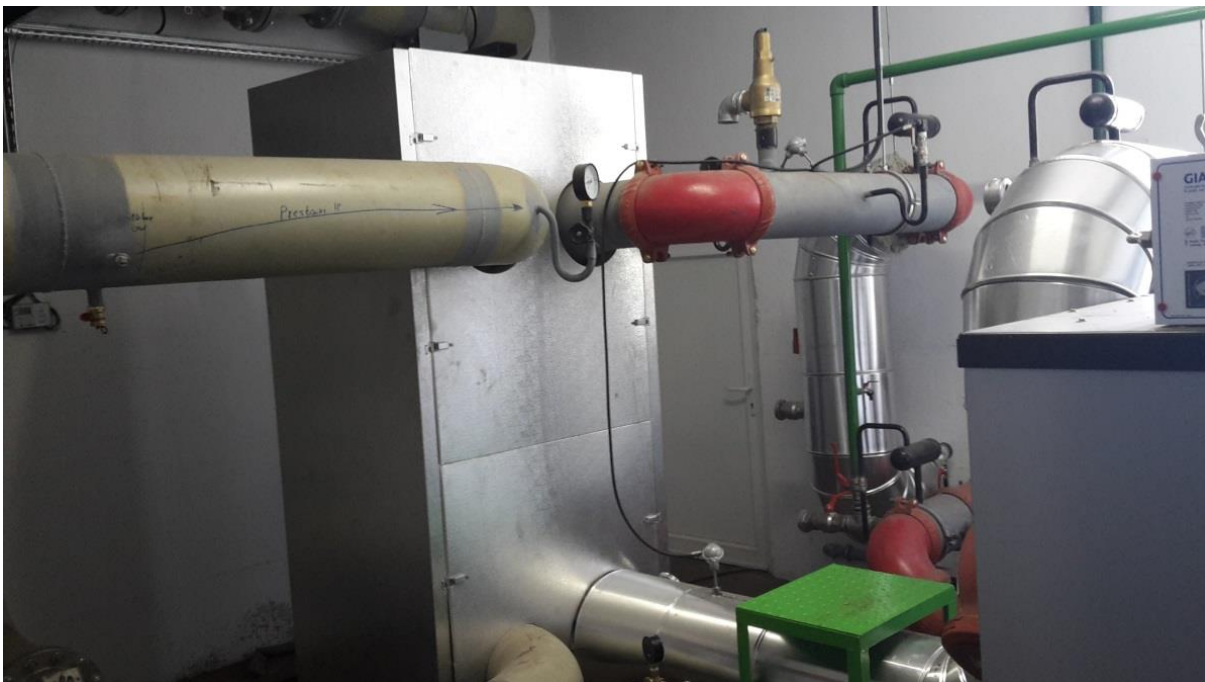
Figure 2: A 4.2 MW heat exchanger near the source of waste heat in SIJ Metal Ravne
