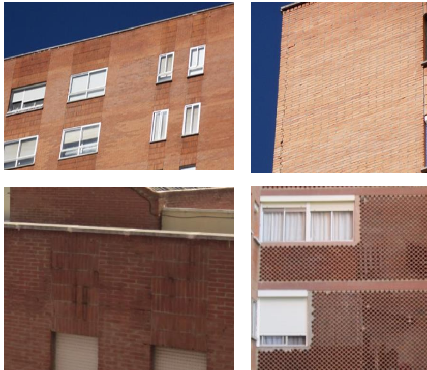
Figure 2. Some of the pathologies in the façades of the buildings (Top left: thermal bridges, top right: fissures, bottom left: efflorescence, bottom right: lattice breakage)
