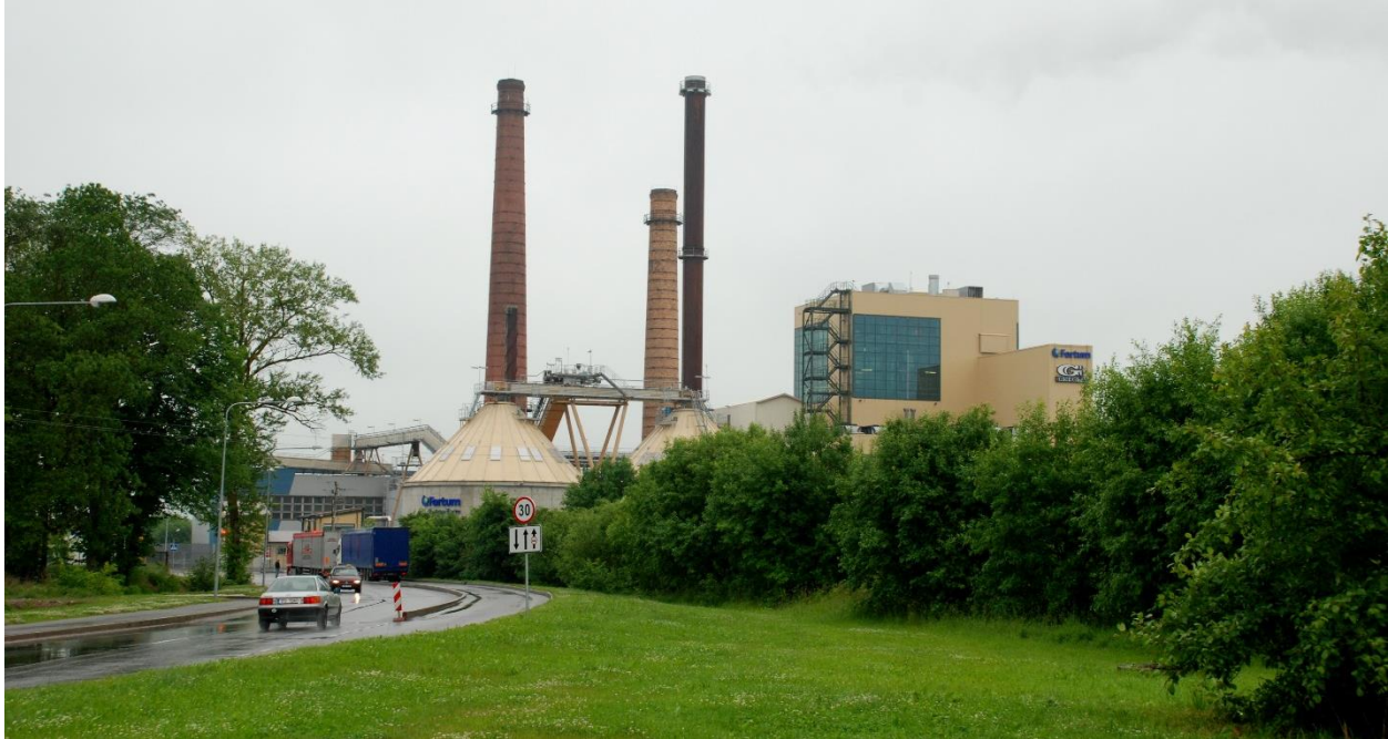
Picture 2. Tartu CHP plant. Photo: Aki Koskinen
