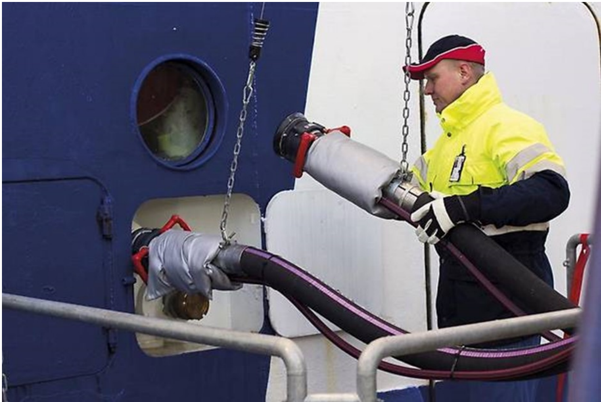
Connecting Stena Danica to the district heating grid. Photo: Göteborgsposten
