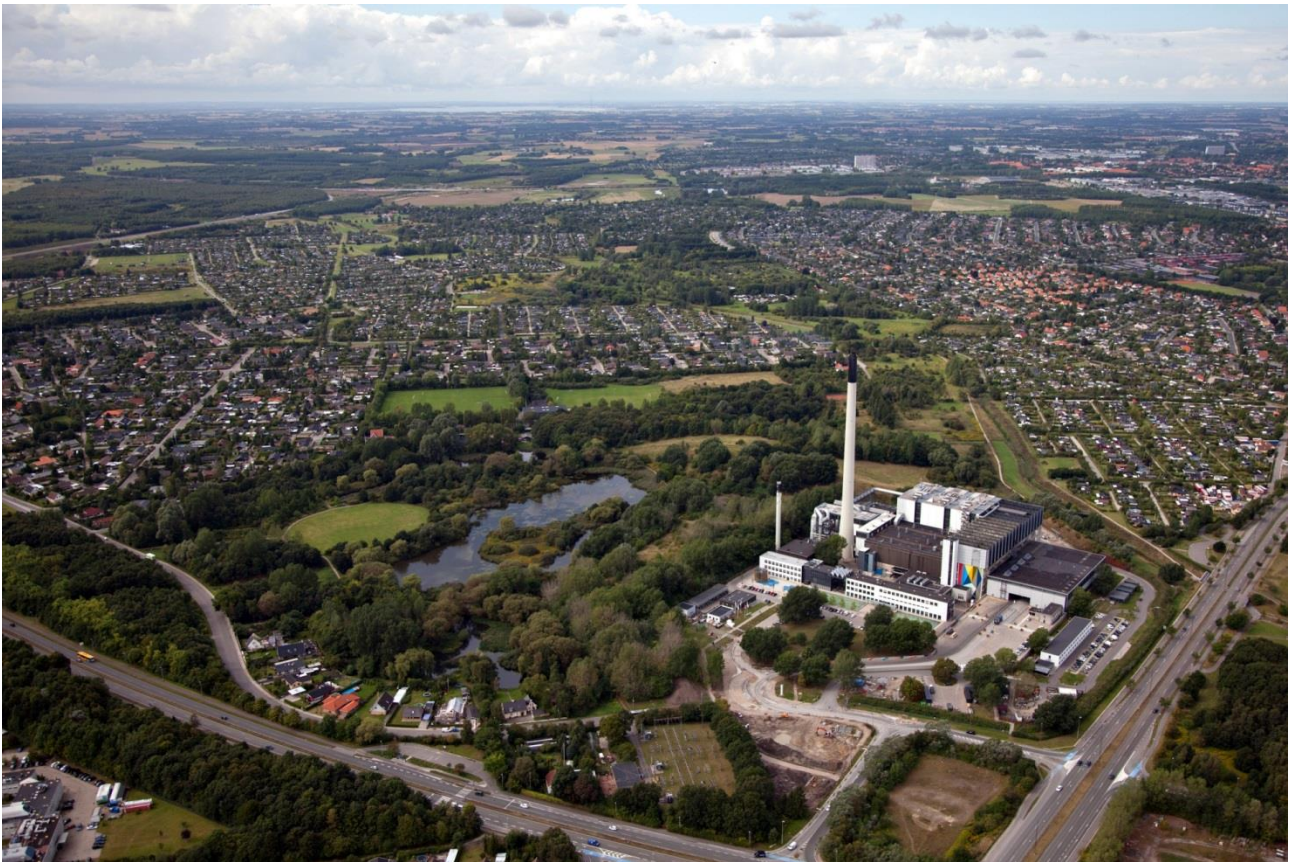
Figure 2 Vestforbrænding, head office and Waste-for-energy plant in Glostrup
