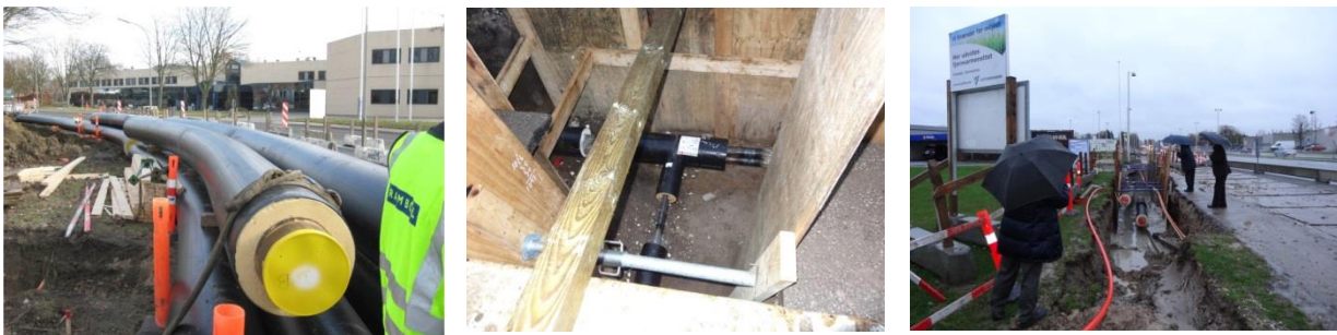
Figure 9 Preinsulated pipes, bended, twin and no-dig
