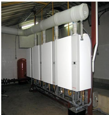
Boiler plant H2D: Type H2D-WTC60-A, product of Weishaupt, thermal capacity 4x60 kW, made of Alumimium, with separate burner and modulated regulation
