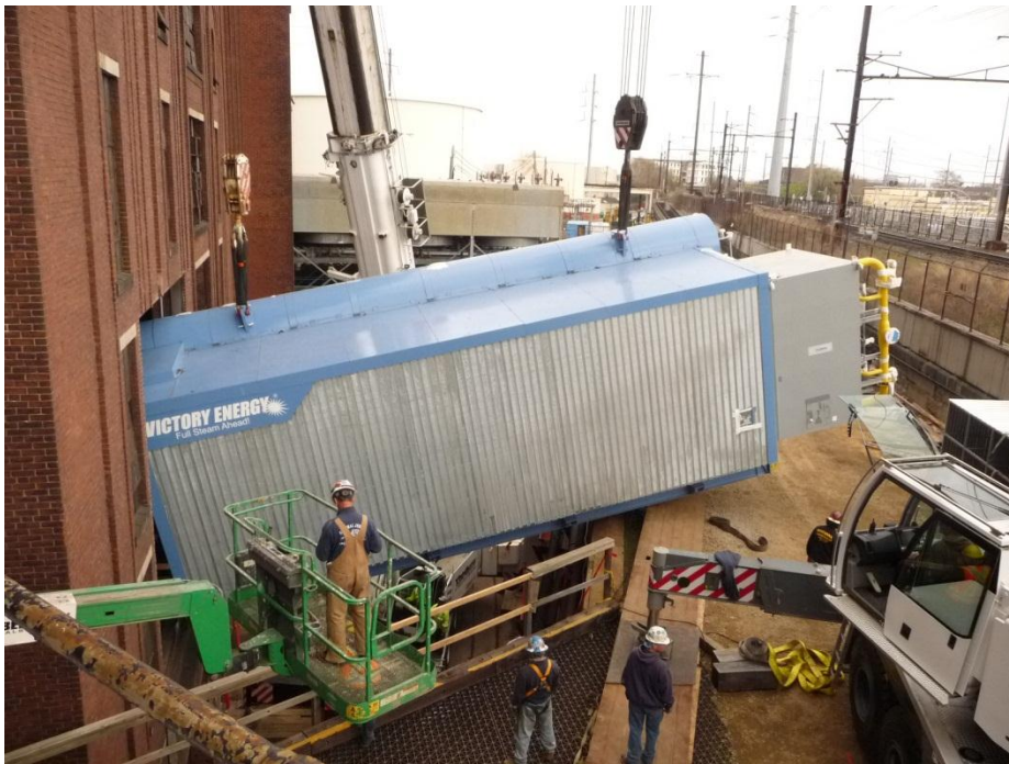
Craning in the Rapid Start Boilers: rigging from 2 levels
