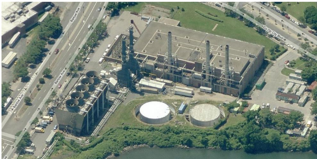
Figure 1. Co-Op City Central Utilities Plant
