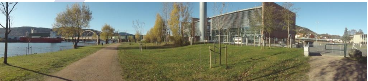
Figure 3 shows the installation in Drammen
