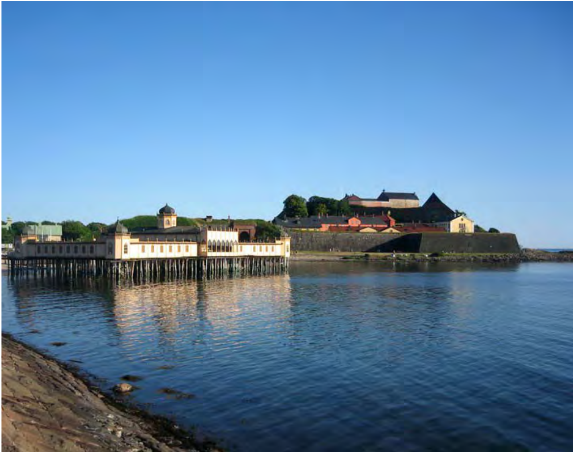
Picture 3. The medieval Varberg Castle was connected to the district heating system in 2006. The beach bathing house remains to be connected.
