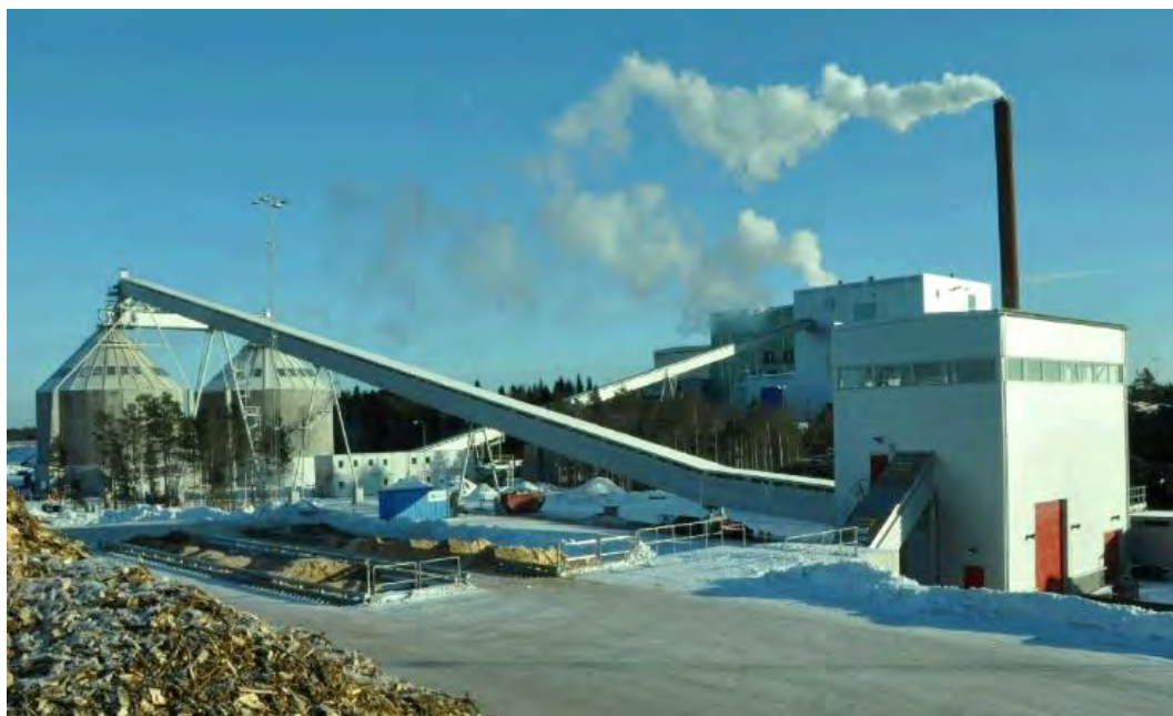
2.8 - Dåva 2 biomass fuelhandling and storage.
