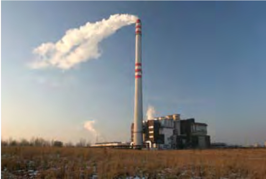
Waste-to-energy plant in Malešice
