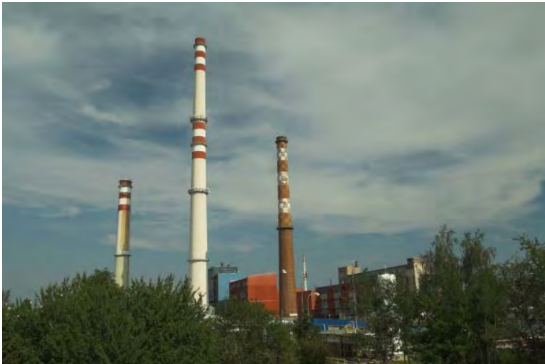
Malešice CHP Plant
