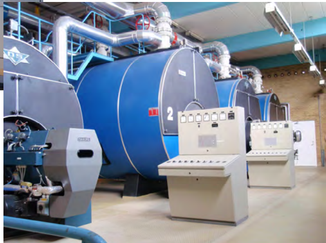
The control panels on the main heating plant.
