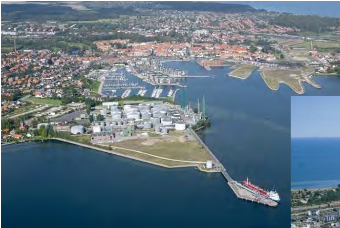
The chemical plant "Koppers Denmark A/S" contributes with surplus heat for approximately 10% of the district heating used in the town of Nyborg.
