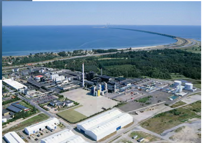
More than 80% of the district heating used in the town of Nyborg is made from surplus heat from the chemical plant "Kommunekemi A/S". →
