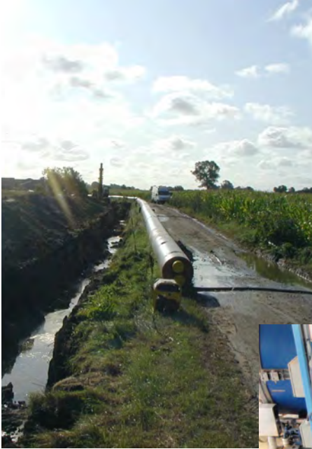
A new transmission line is under construction.
