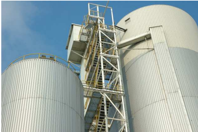
Modern flue gas desulphurisation system is one of many ways of limiting noxious emissions to the environment.
