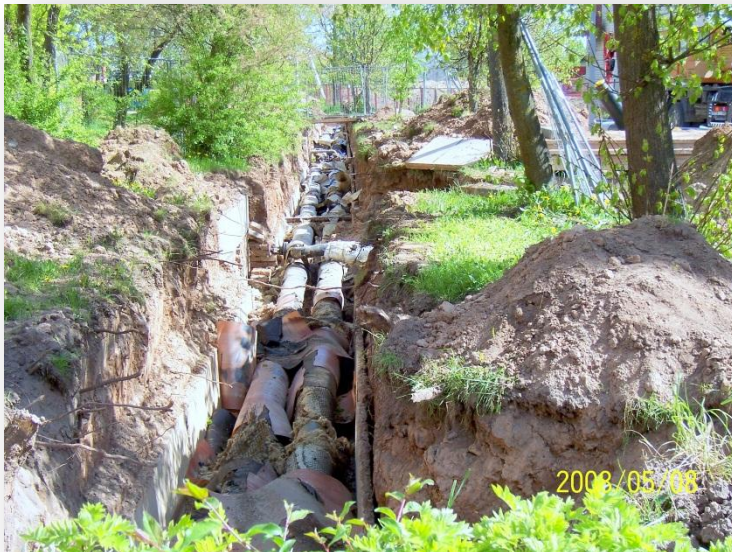
Picture 5. Status of heat transmission networks during reconstruction.
