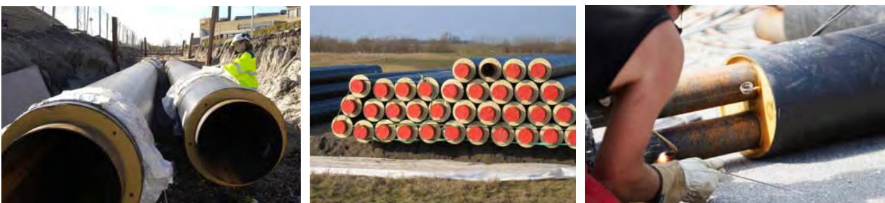
Picture 3. From left: Large distribution pipes in Malmö, pipe storage for ongoing distribution project, pipes are being welded together. (Photo: E.ON)
