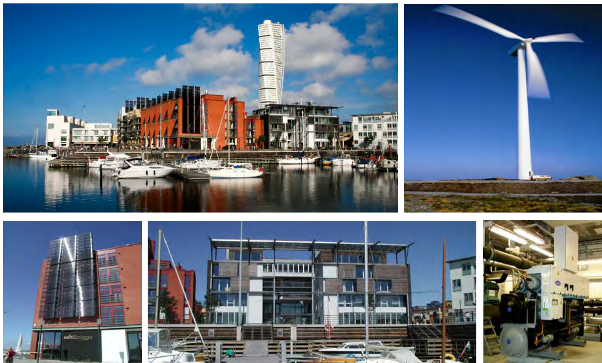
Picture 5. The Bo01 area in the Western Harbour is supplied by the unique energy system “100% locally renewable energy”, designed and constructed by E.ON. The systems’ components are: wind power, solar cells, solar panels and an aquifer in cooperation with a large heat pump. (Photo: E.ON)
