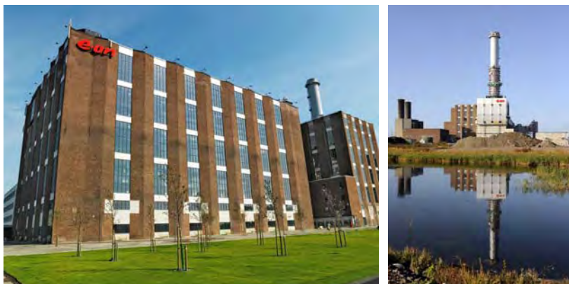
Picture 1. High efficient CHP plant Öresundsverket, inaugurated 2009. (Photo: E.ON)
