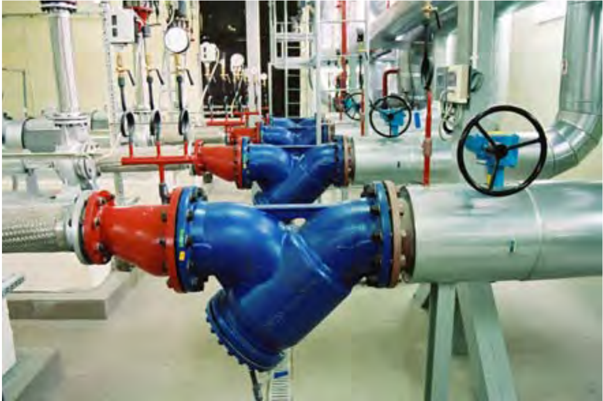
Pumping station Wola Duchacka in Kraków
