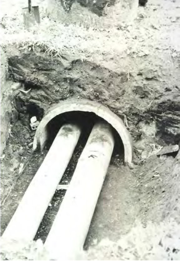
Old and new heating pipelines
