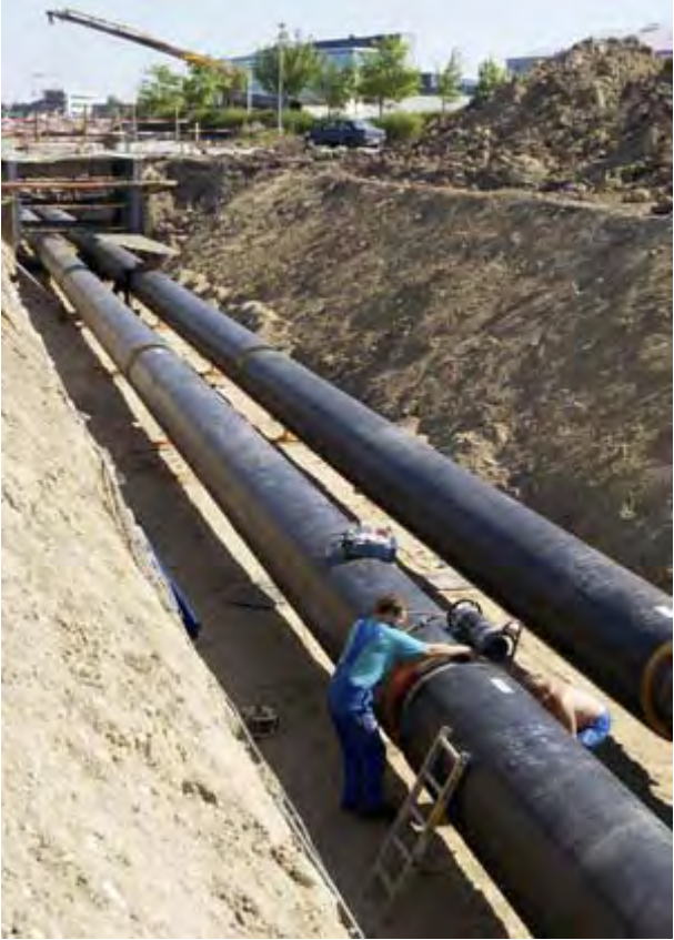
Old and new heating pipelines
