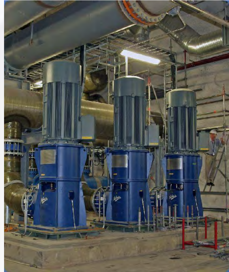
The purified sewage water pump
