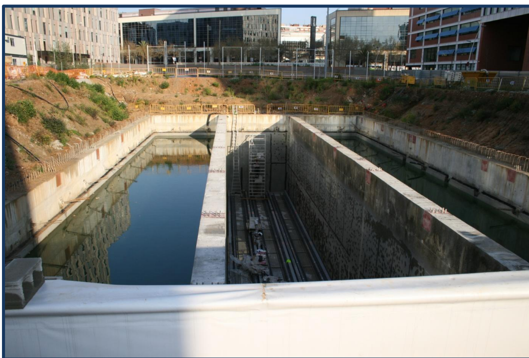
Fig. 14: Ice tank construction.
