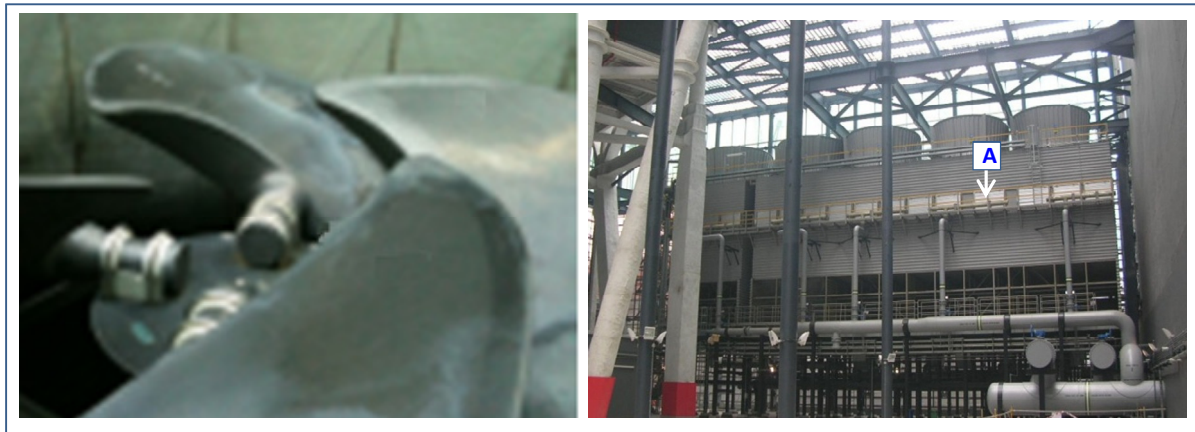
Figure 10. Special provisions for cooling towers: (Left) Ultra-low noise fans. (Right) Plume abatement coils A
