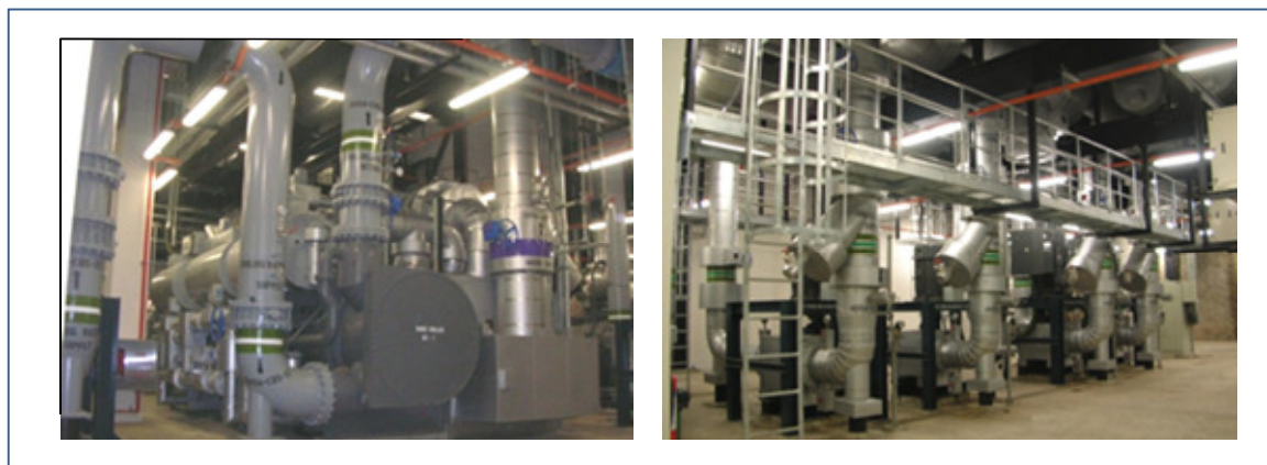
Figure 4. View of machinery in Plant1 : (Left) 10MW Brine Chiller. (Right) Distribution pumps
