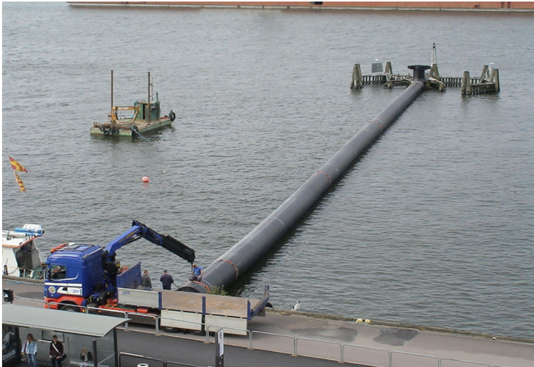
Picture 5, the free cooling lake water intake
