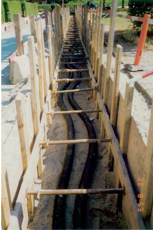
Illustration 2: District heating pre-insulated S-curve piping
