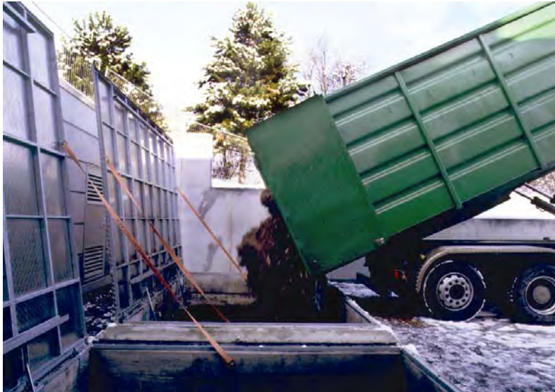
Wood chip delivery and transport in the heating plant
