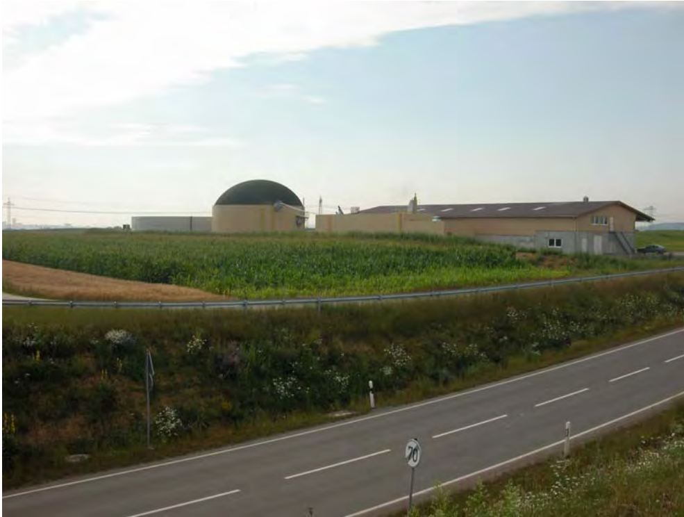
The Biogas plant in Sachsenheim
