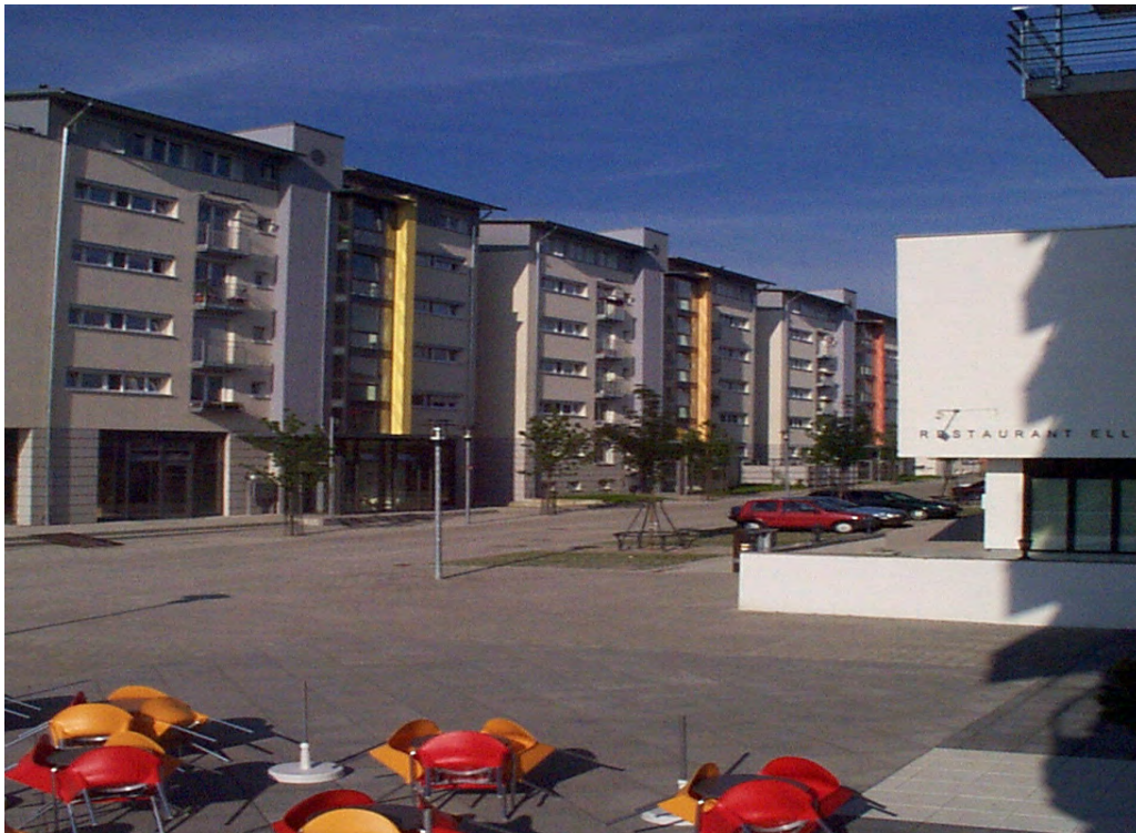
Low energy multi family houses in “ Kreuzäcker/Ellental “ in Bietigheim-Bissingen,
