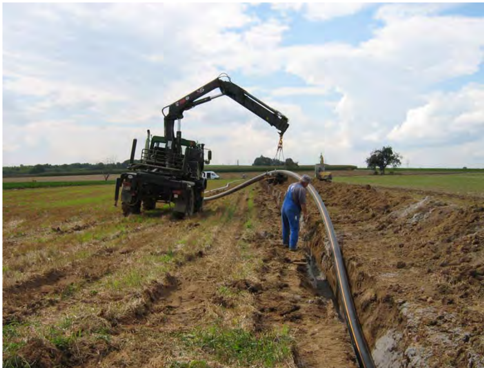
Construction of the Biogas-pipeline
