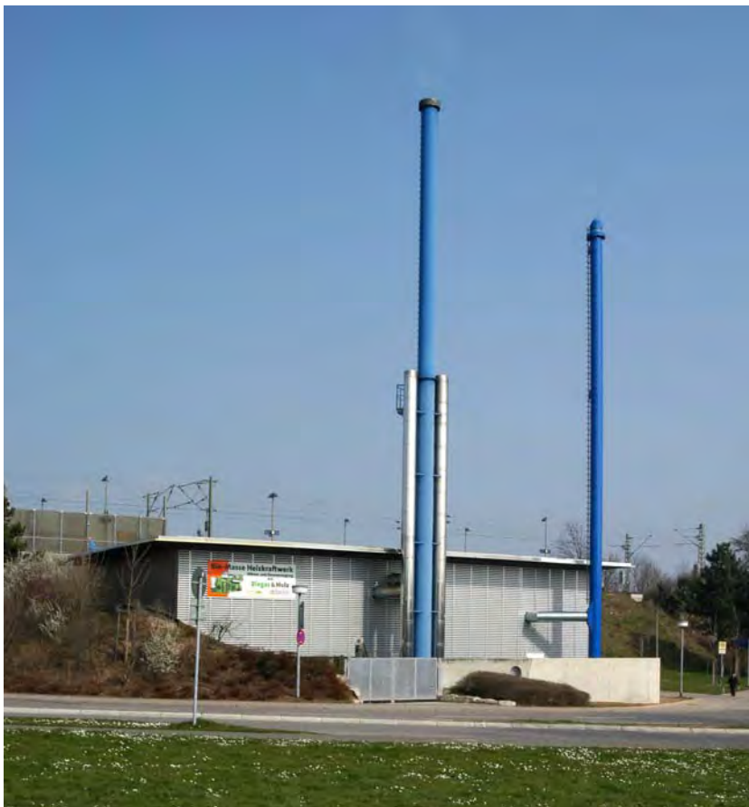
Central biomass heating plant Kreuzäcker/Ellental
