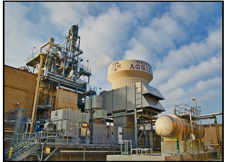
Gas Turbine Generator 1 (GTG1) 34 MW 45,600 HP
