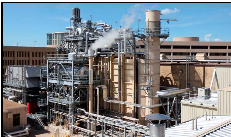
Heat Recovery Steam Generator (HRSG) 600 psi, 210 mlb/hr
