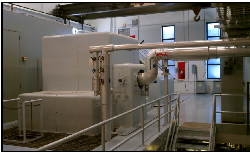
Steam Turbine Generator 4 (STG4)
