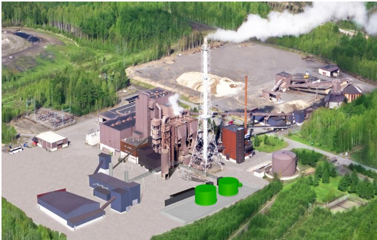
Picture 2. Trigeneration plant in Joensuu.
